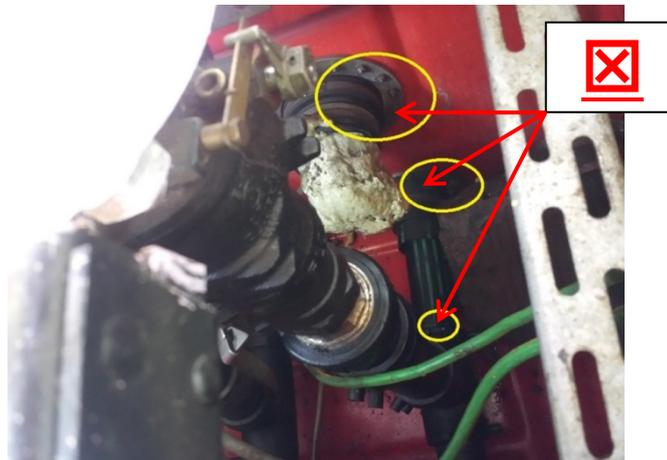
**Figure 5: No bonding across composite piping of fuel dispenser**
